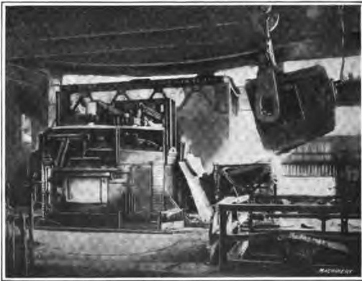
Fig. 2. Twenty-five ton Héroult Furnace receiving Charge of Molten Metal
